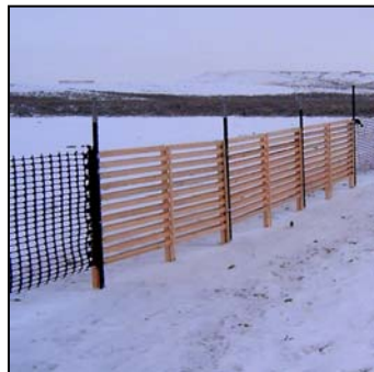
Figure 7. Hollow Frame Fence Line.
