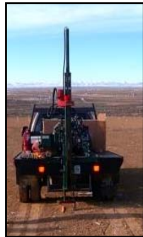
Figure 10. Soil Moisture Access Tubes Installation.
