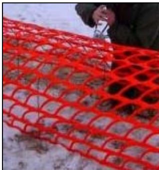
Figure 6. Constructing Snow Snake Fences.
